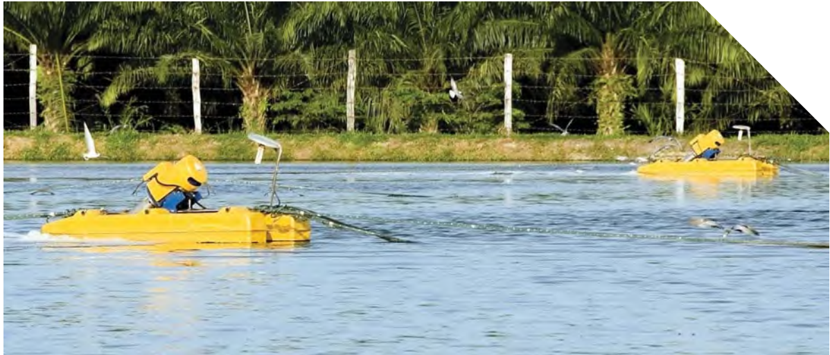
Instalasi Pengolahan Air Limbah, BSP (Bunut - Sumatera Utara) | Waste Water Treatment Facilities, BSP (Bunut - North Sumatra)
